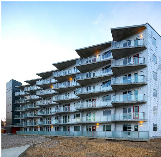
Parkdale ONE. Photo courtesy of GEC Architecture, 2018
